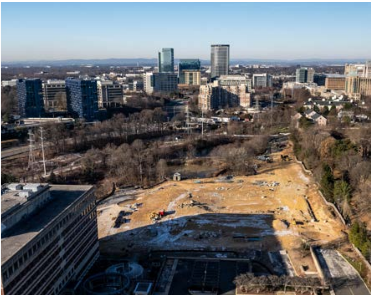
The American Dream Way project shortly after groundbreaking in 2024. The upscale housing project was set to be completed the end of 2026. Land development is a hot topic in Reston, with major projects underway and proposals for more on the rise. Photo by Benjamin Burgess
