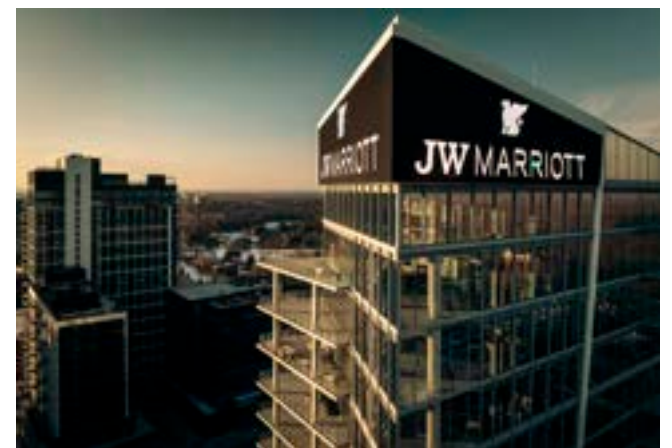
Since its installation this fall, the JW Marriott sign has concerned some residents in the area with its brightness.
